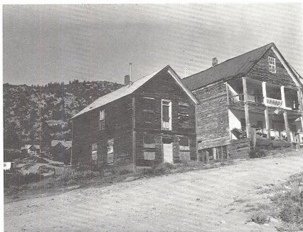
FIGURE 2-30. Old Hotel Annex (Block 4, Lot 81). Present use is dwelling.
